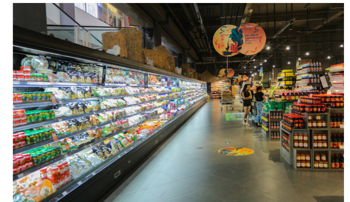
S-store /C-store /supermarket Area: 1000m 2 -5000m 2 Cabinet Temp.: -1°C ~ 10°C OAT: -30°C ~ 48°C
